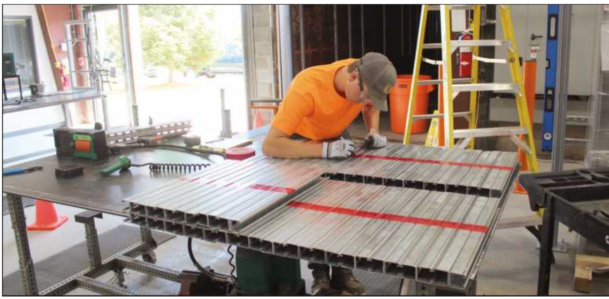
IBEW LOCAL 665 apprentice Ryan Lay marks up conduit strut hangers while working in the new shop at the Superior Electric Great Lakes Co. in Lansing. They will be installed at the Ultium Battery Plant project under construction several miles away.
